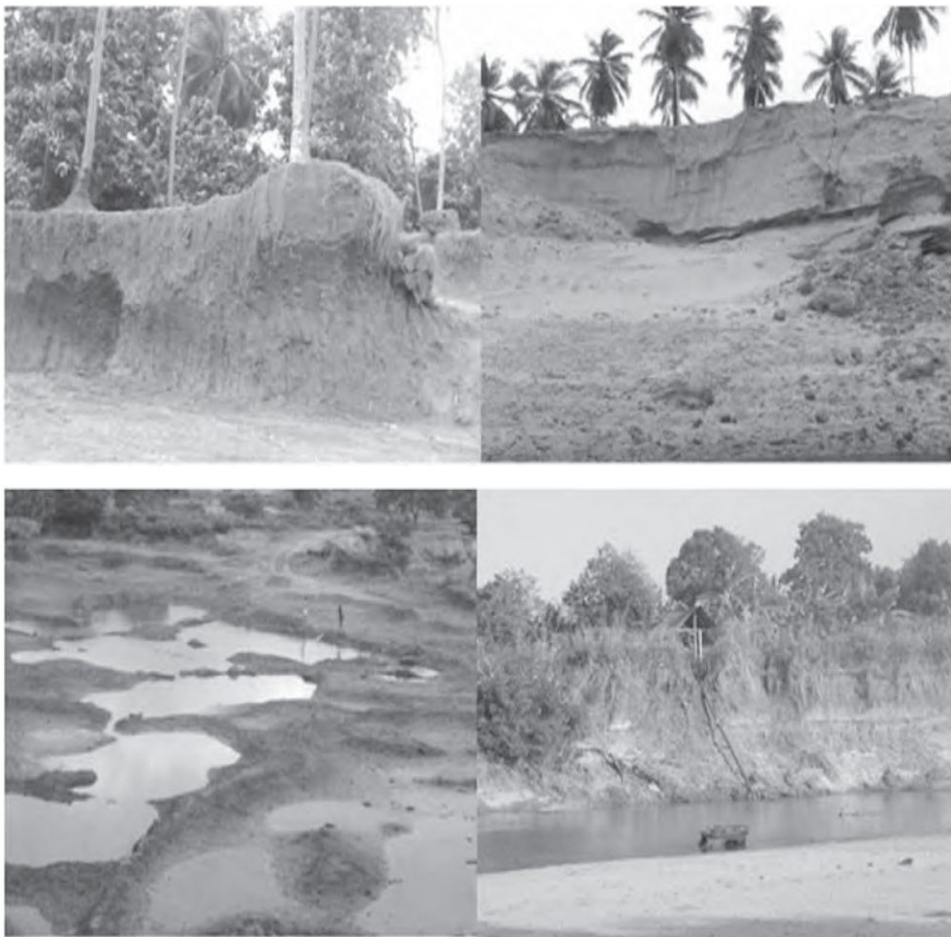
Damage to banks and riverbed (Photo Courtesy : Ranjith Ratnayake)
