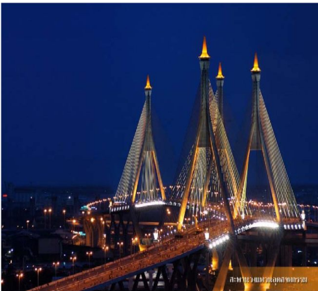
(Industrial Ring Road Bridge)
